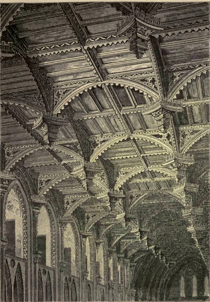
ST. DAVID'S CATHEDRAL. ROOF OF NAVE.
